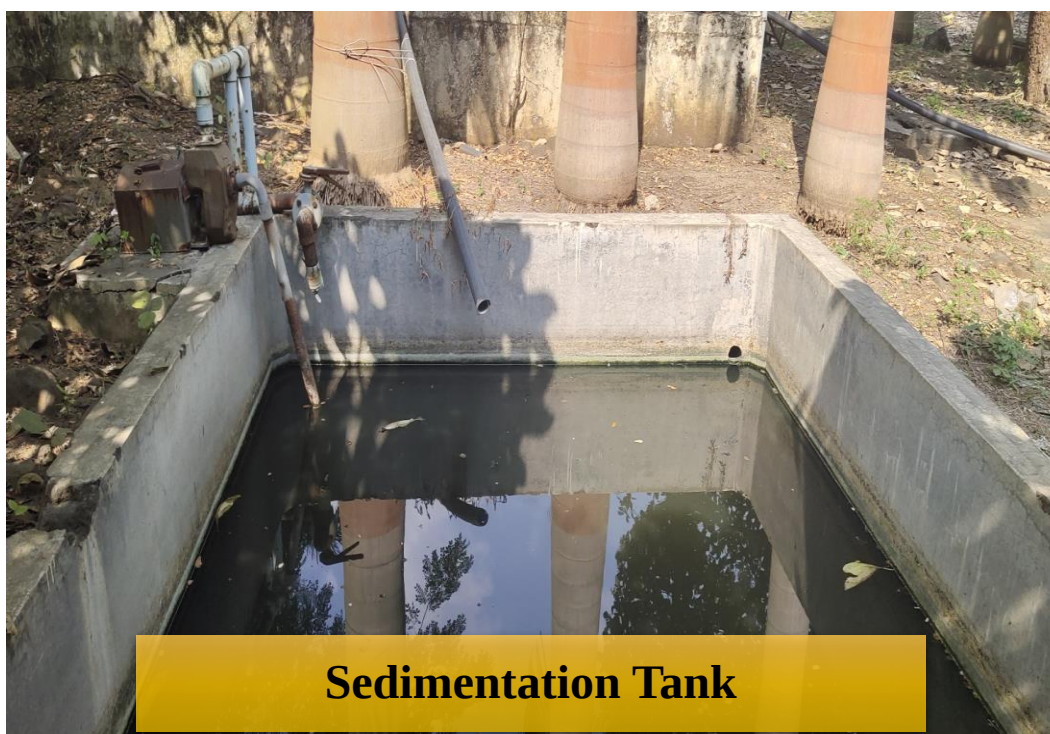
Photograph No. : Sewage Treatment Plant
