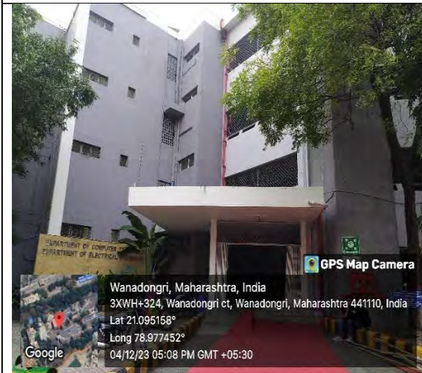
Computer Tech. & Electrical Engg. Department
