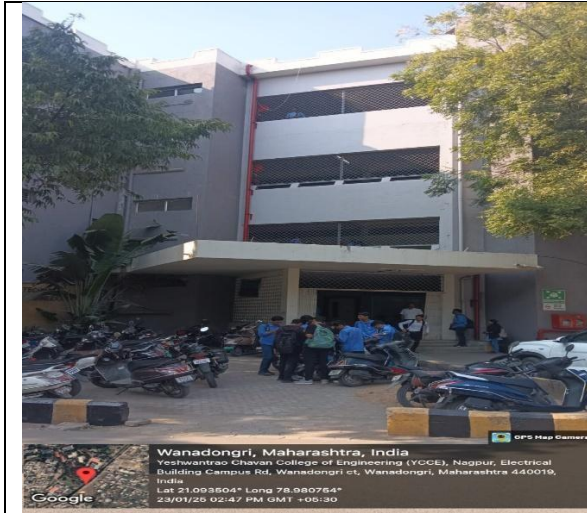
Computer Tech. & Electrical Engg. Department
